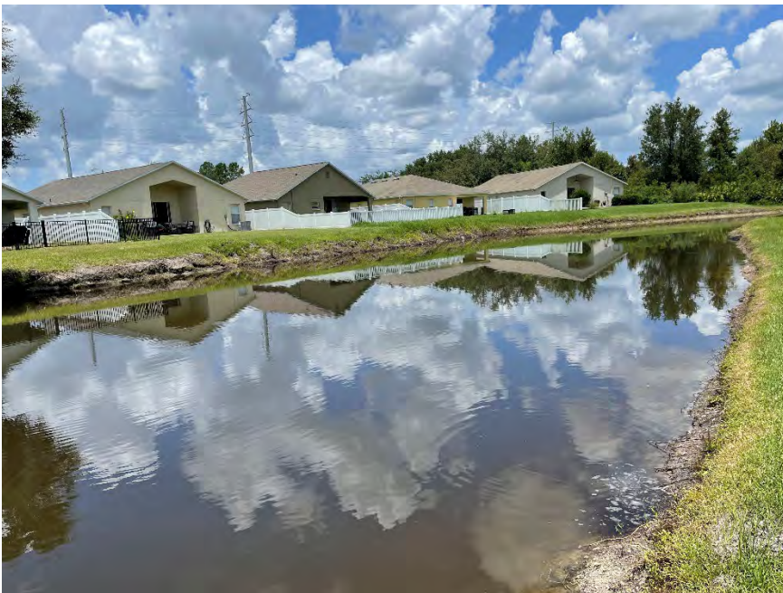
Photo showing the overall condition of the pond bank. Approximate exposed pond bank is 350 feet.
